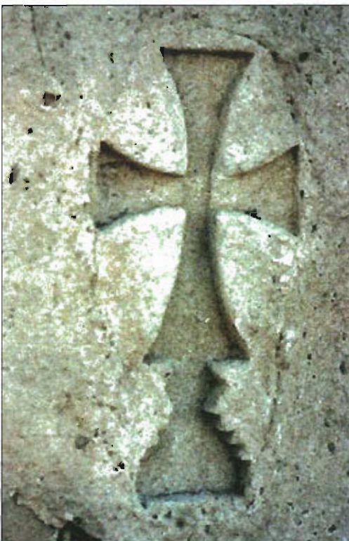
Cross design in a doorway of the church. This recessed outline may have originally contained a stone or wooden cross
