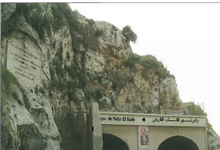
Tunnel entrance to Nahr el-Kalb, Lebanon
