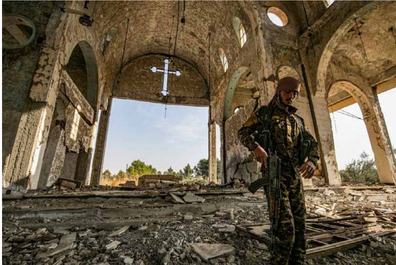
A member of the Khabour Guards (MNK) Assyrian Syrian militia, affiliated with the Syrian Democratic Forces (SDF), walks in the ruins of the Assyrian Church of the Virgin Mary, which was previously destroyed by Islamic State (IS) group fighters, in the village of Tal Nasri south of the town of Tal Tamr in Syria's northeastern Hasakah province on Nov. 15, 2019.
