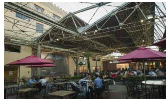
The original steel roof beams from the tire and rubber factory that later became the Citadel Outlets are still visible above the mall's food court in Commerce, California.
